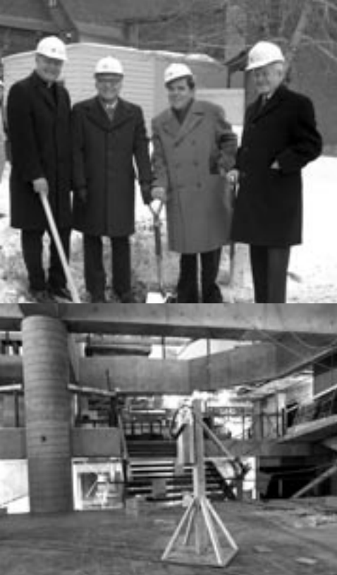
Top: Groundbreaking ceremony, January 13, 1972. 168 Bottom: Construction in foyer of Fauteux Hall, May 1973. 174
