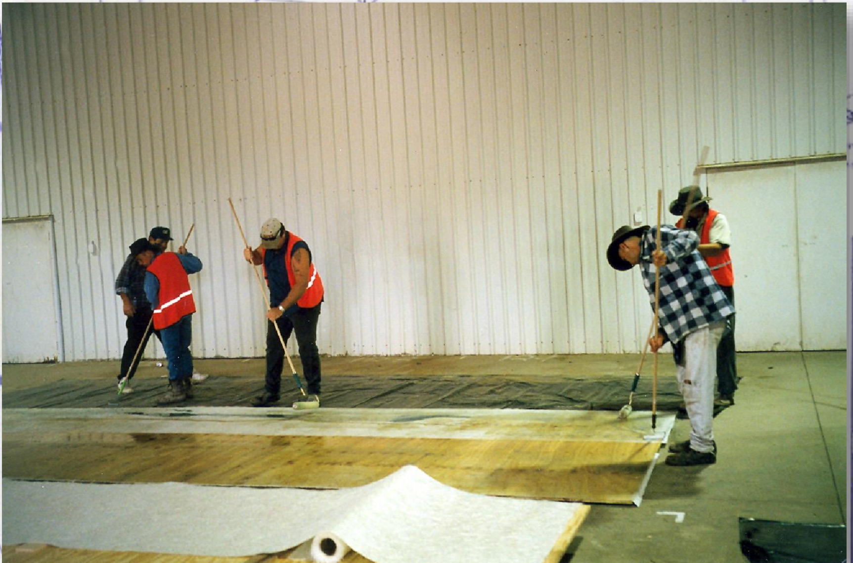
Two layers of fiberglass is applied to plywood sections.
